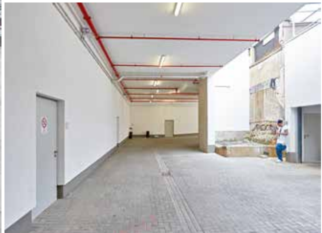
External doors are located in the partially roofed inner courtyard of the delivery area.
