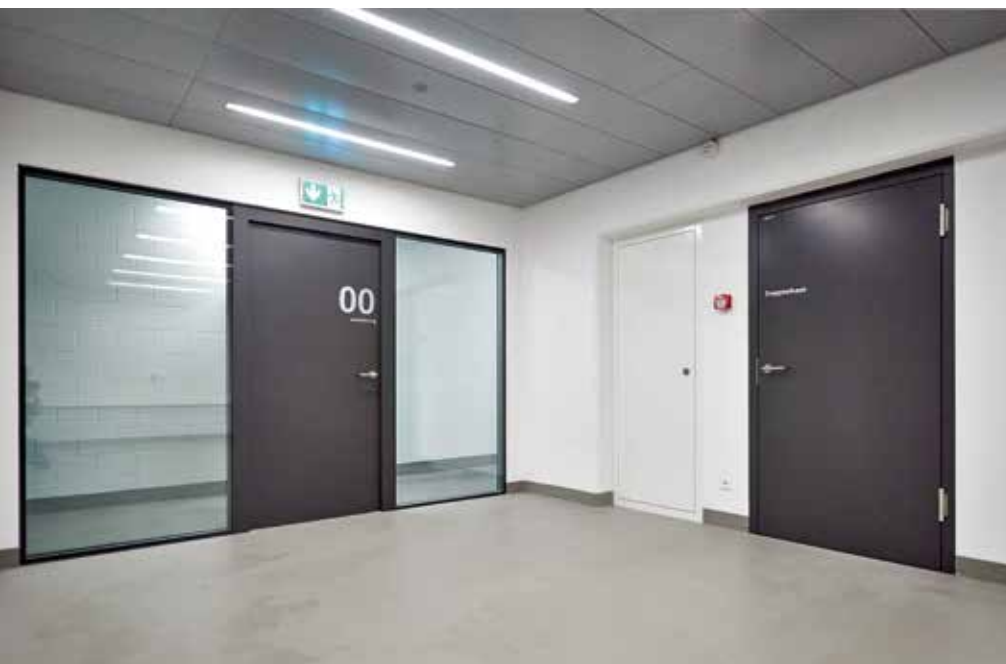
The panes are mounted flush-fitting with the frames.
