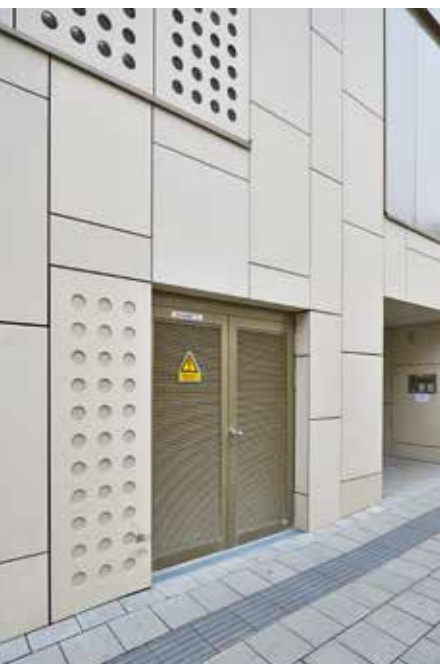
External door with ventilation slats. Double-leaf fire-rated and smoke-tight doors protect the escape routes to the outside.
