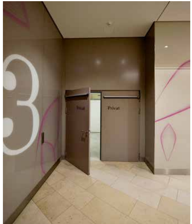
Double-leaf fire-rated and smoke-tight door in the Minto.
