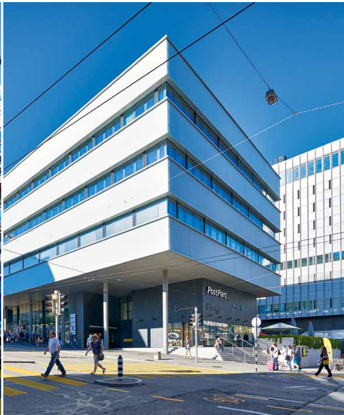
The retail and dining areas in the PostParc were designed in such a way as to avoid mono-structures.
