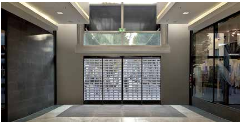
Shops are securely closed by the combination of automatic sliding door and rolling grille.
