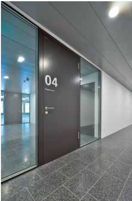
Fire, smoke and acoustic rated doors made of timber by Schörghuber were used throughout the entire building – including the basement and underground car park.
