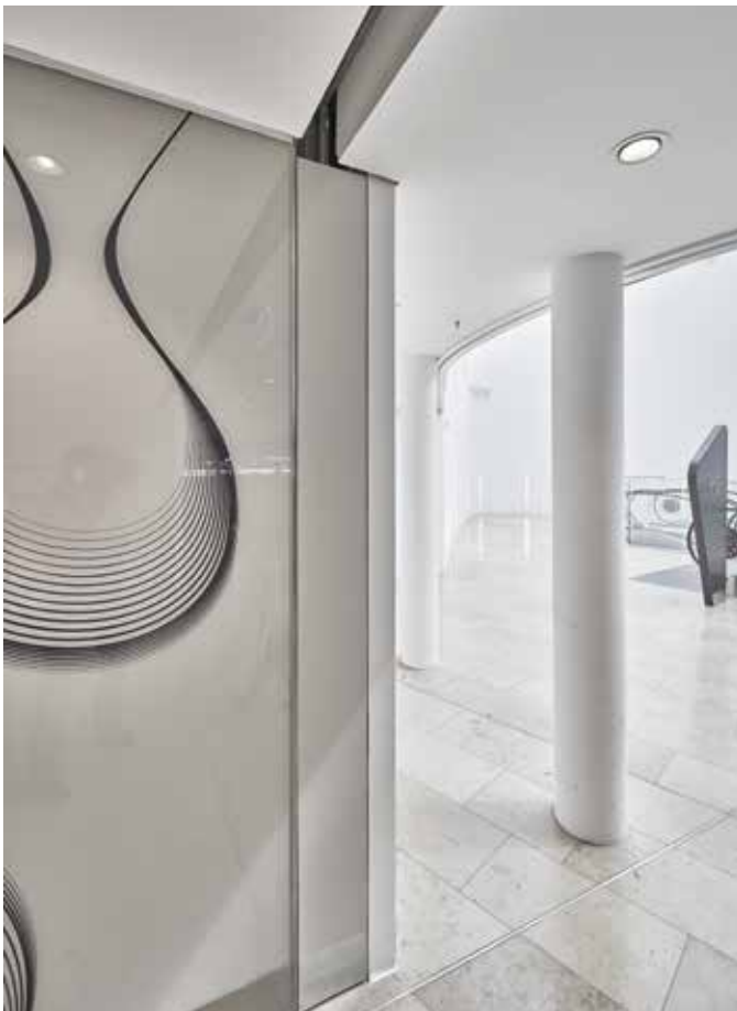
The fire sliding door is hidden behind a recess flap.
