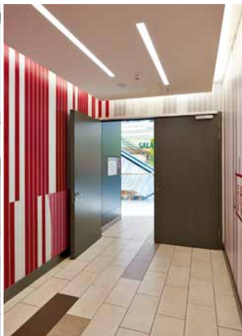
External door with ventilation slats. Double-leaf fire-rated and smoke-tight doors protect the escape routes to the outside.
