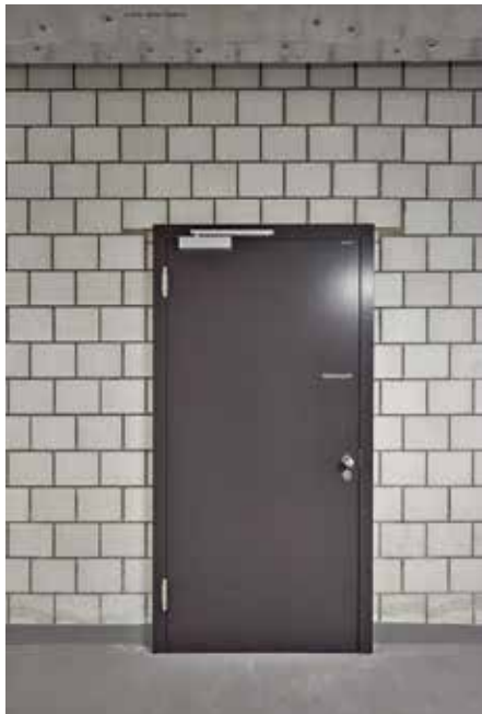
Fire, smoke and acoustic rated doors made of timber by Schörghuber were used throughout the entire building – including the basement and underground car park.
